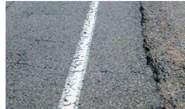
EXISTING ROAD PAINT
